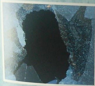
Windows break at level 5
